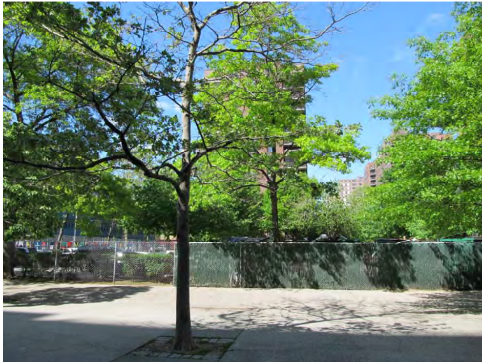
5. Looking North at the subject site from West 97 th Street.
