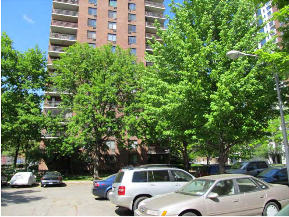
3. Looking North from the subject site.
