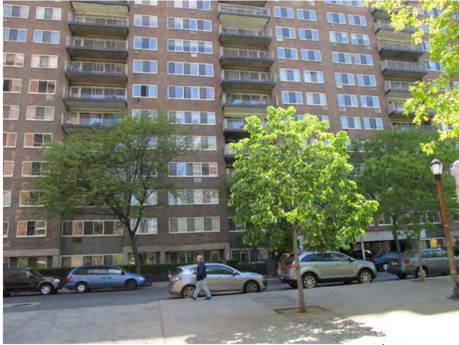
1. Looking South from the subject site towards 120 West 97 th Street.
