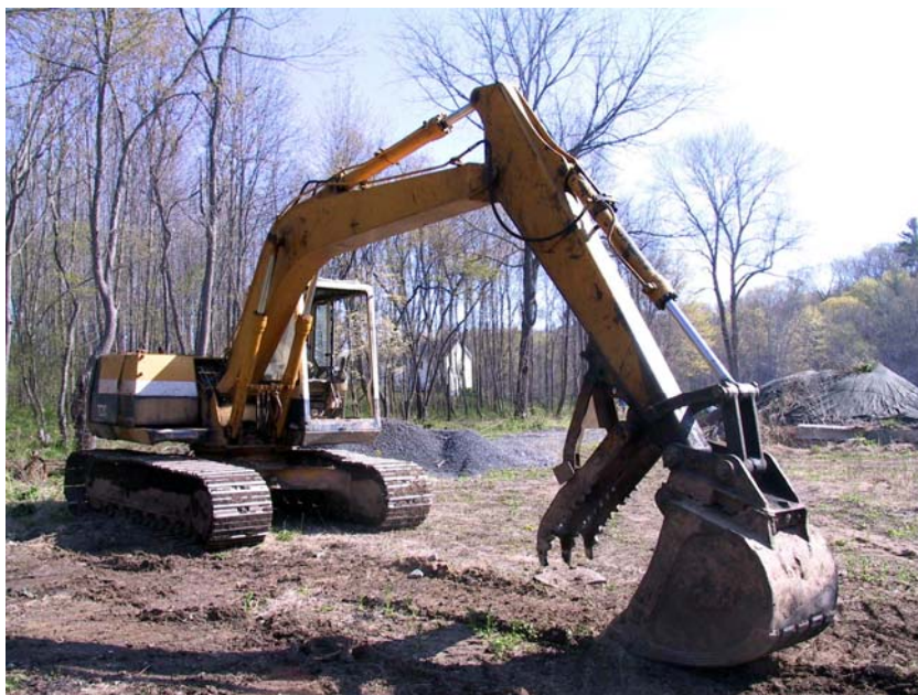
Photo 1. The hydraulic excavator that was involved in the incident.
