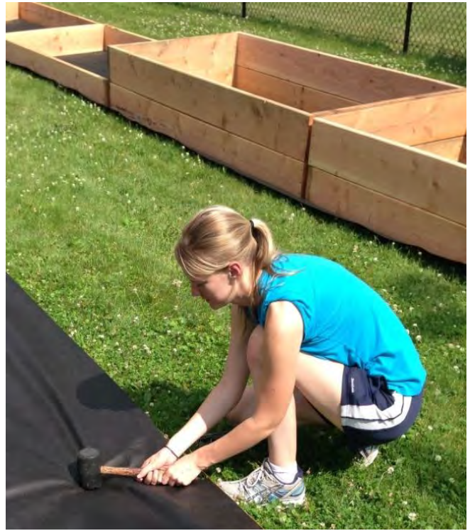
Figure 4. Using a mallet to pin landscape fabric
