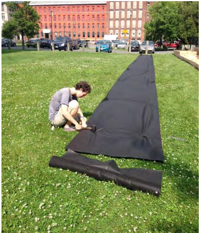
Figure 5. Landscape pins placed 3 – 5 feet apart
