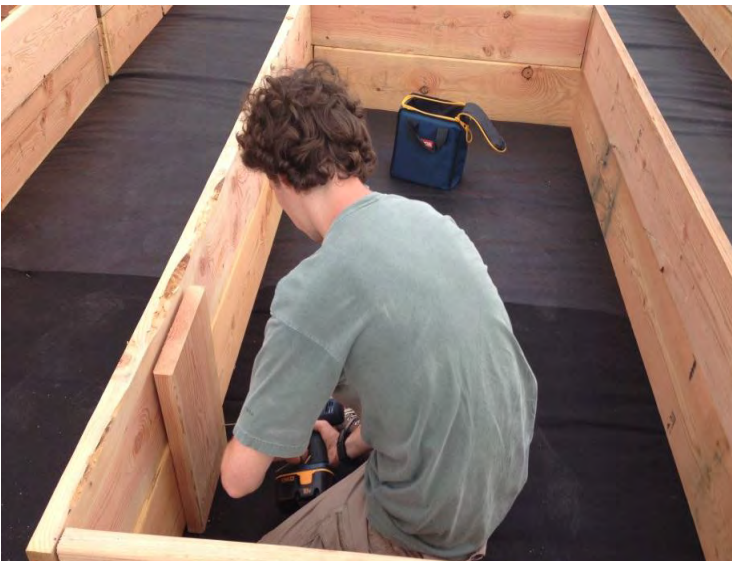
Figure 11. Putting a brace on a double box. (This photo and Figure 13 are from a garden where we covered the paths between the boxes with landscape fabric, too. They would later be covered with gravel, stone dust, or other material.)
