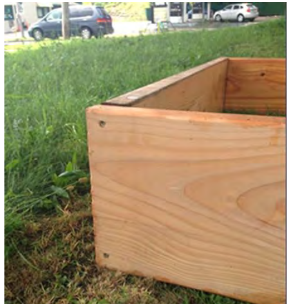
Figure 10. Placement of two screws in corner (four screws will be needed per corner)
