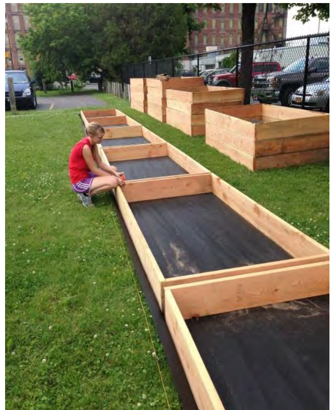
Figure 12. Lining up the boxes
