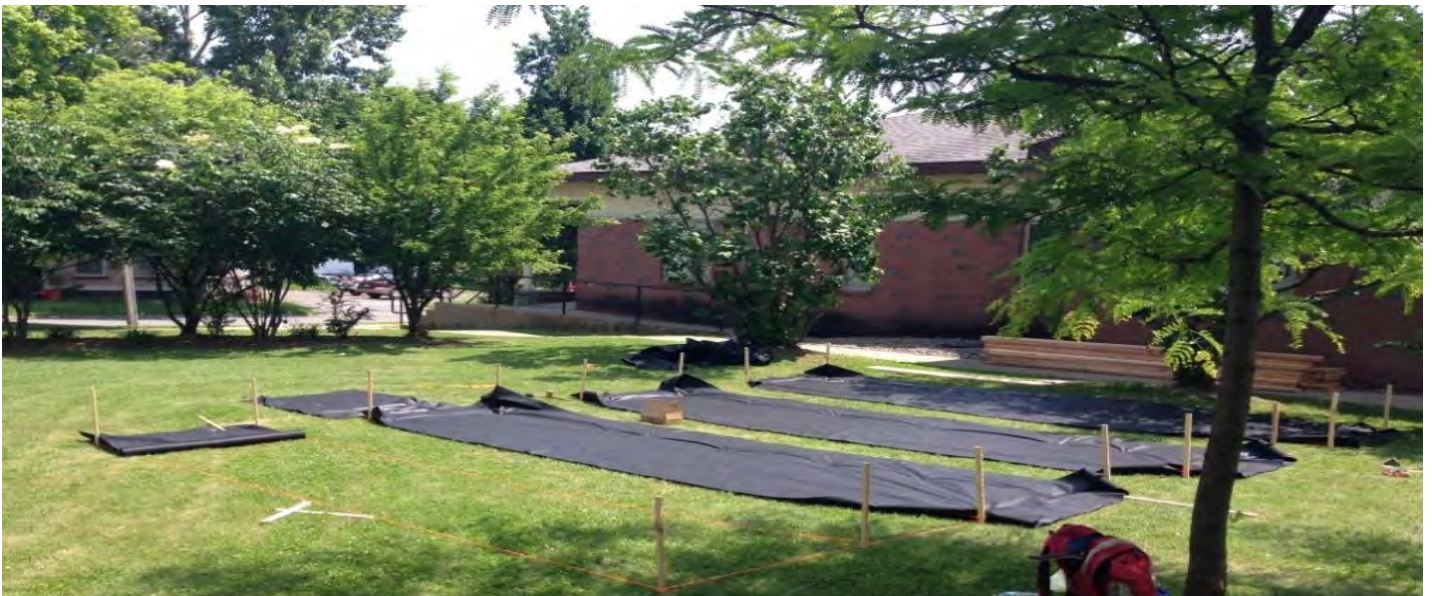
Figure 7. Garden site development in progress
