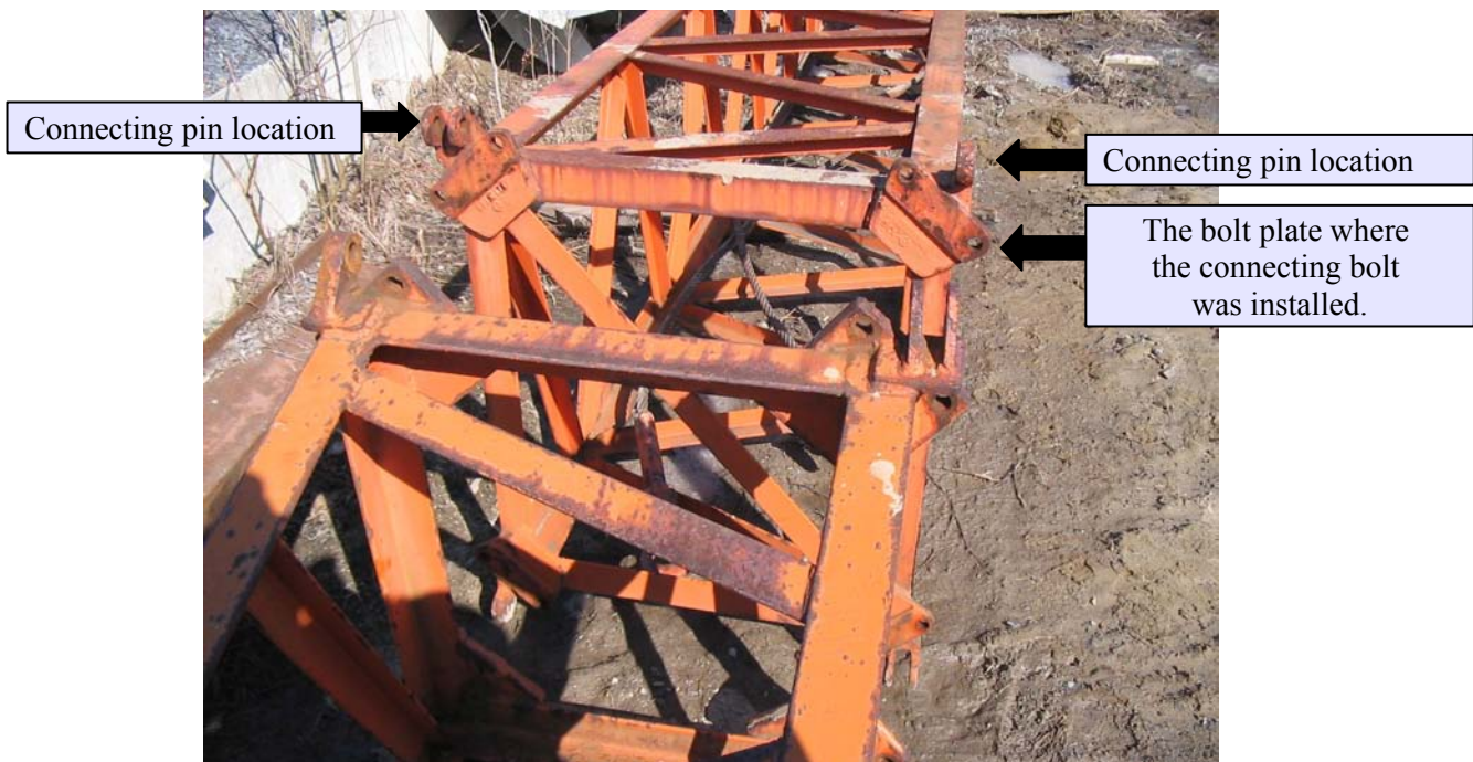
Photo 1. The photo illustrates the connecting ends of the two adjacent boom sections. There were eight bolts and four connecting pins connecting the two boom sections (Photograph courtesy of OSHA).
