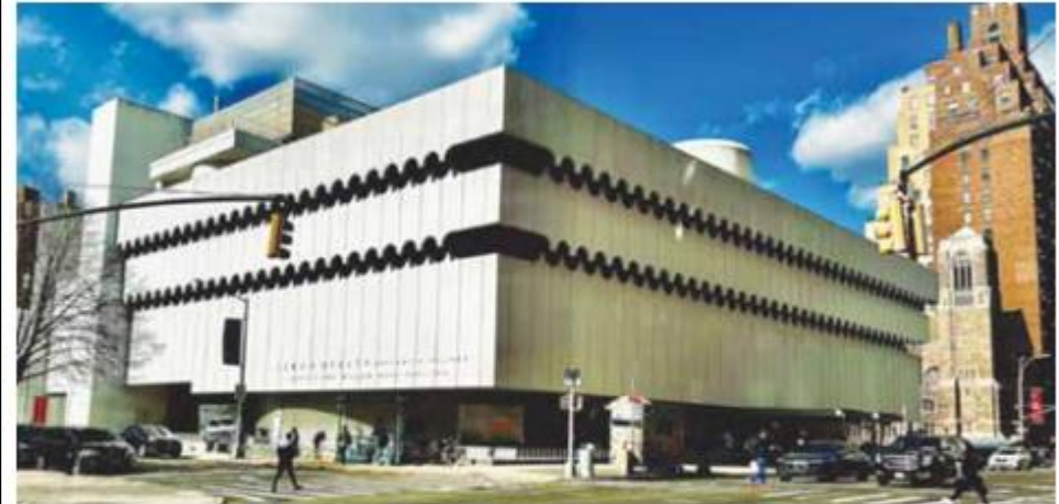
THAT WHITE BUILDING AT SEVENTH AVENUE is the Lenox Health Greenwich Village facility since 2014. Credit: Brian J. Pape, AIA.
